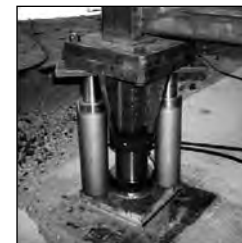
Contractors called on the brute force of Simplex R5513 cylinders to lift and position highway ramps in San Diego. The Simplex 50 Series power units provided the power and control in this rough outdoor application.
