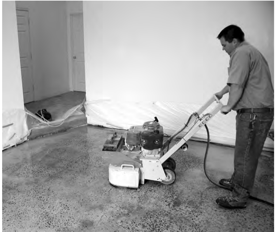
Dual-Disc Grinder will grind approximately 350-500 sq. ft./hr. at 1/32" with EDCO Dyma-Serts.
