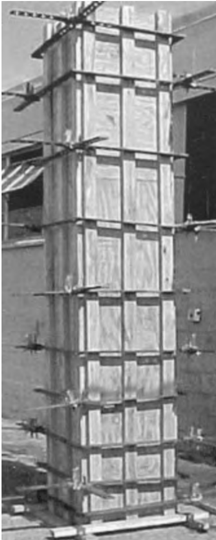
Typical 24" x 24" column form – Ready to pour.
