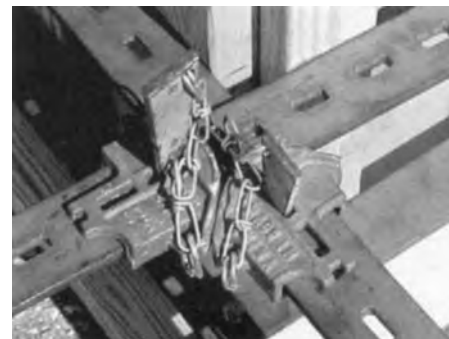
Wedges are used to tighten Column Clamps.
