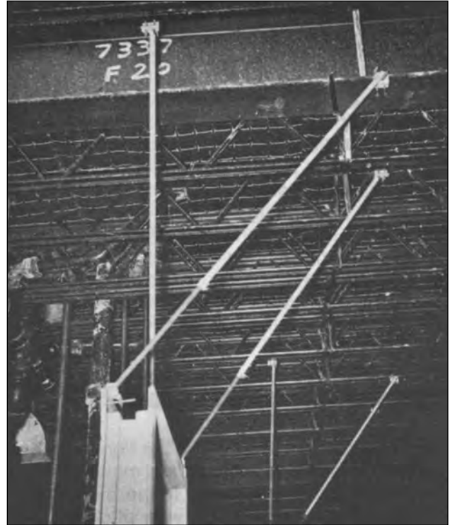
Buck-Ups clamped to bar joists and I beams.
