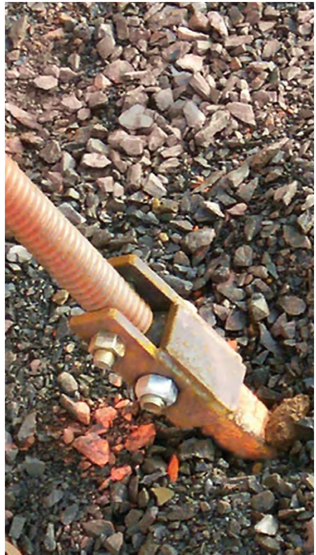
INCORRECT Brace-to-HGA Connection
